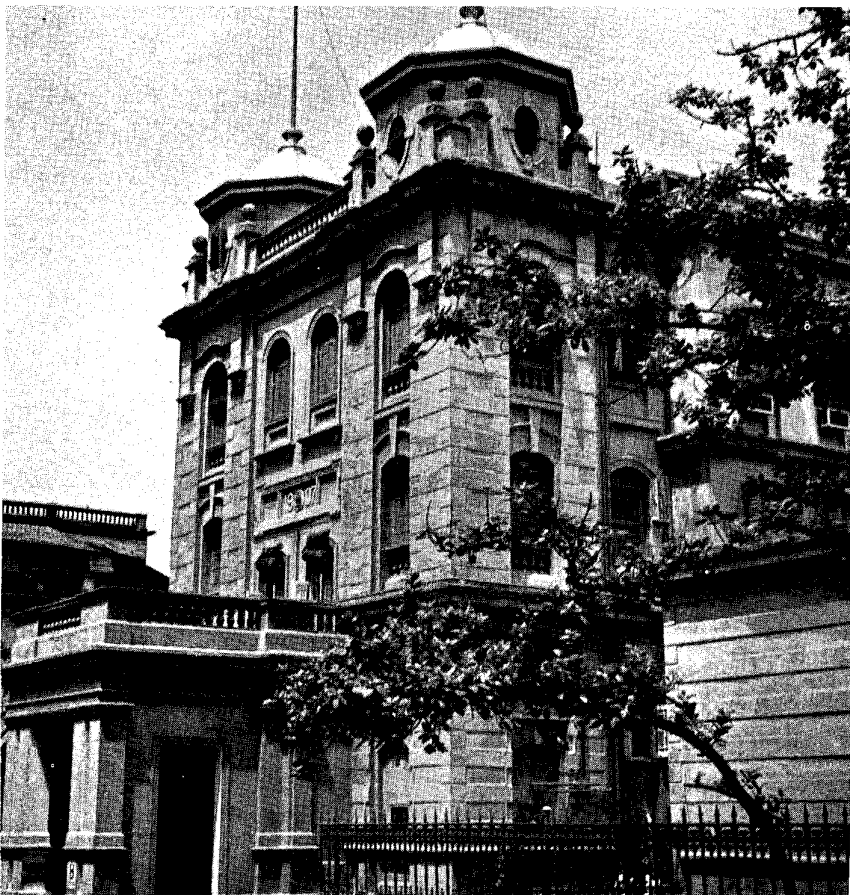
The Andrew Yule building at 8, Clive Row in Calcutta.
